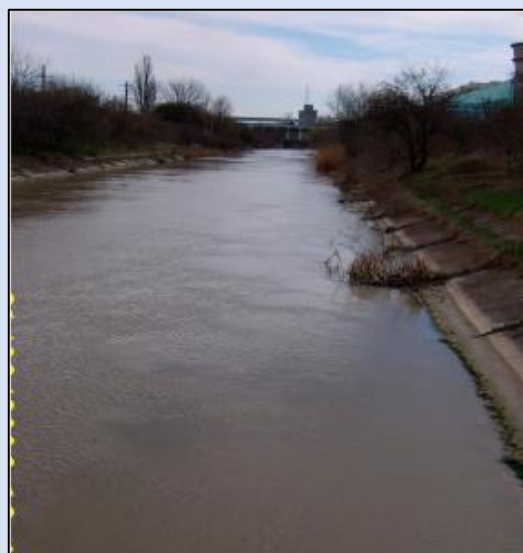
Figure 11.4: CFPP process water inlet channel to Jiu River Romania
